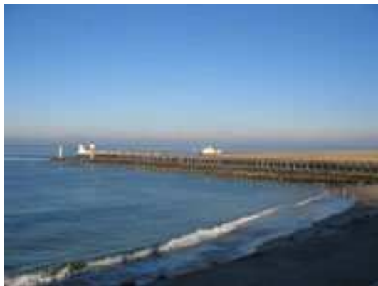
Impact of the north dyke: strong accretion to the north, erosion to the south
